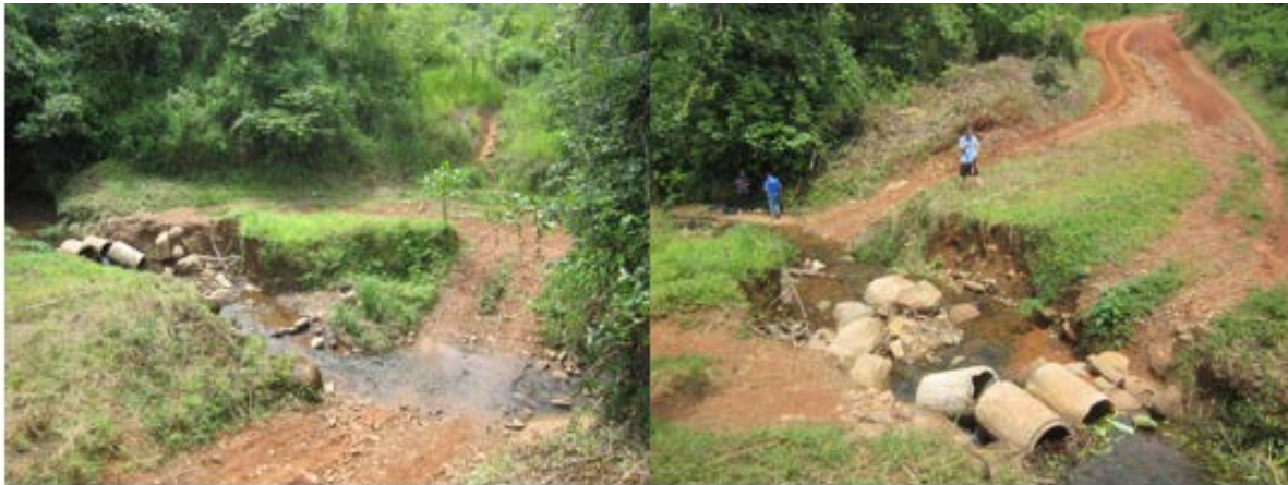
Figure 6. Roadways leading into project location (a) looking north, (b) looking south
