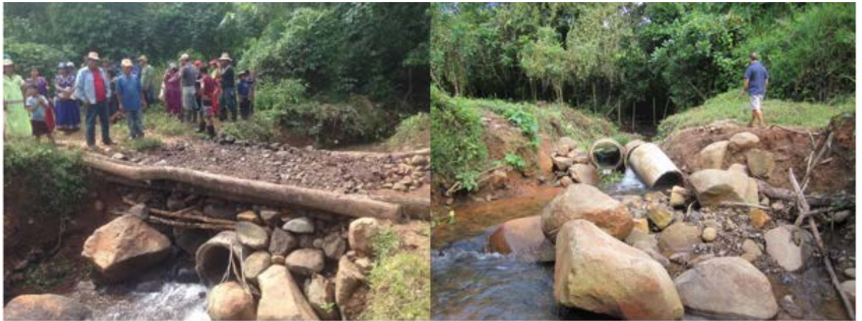
Figure 7. Past attempt at a solution for the problem stream crossing
